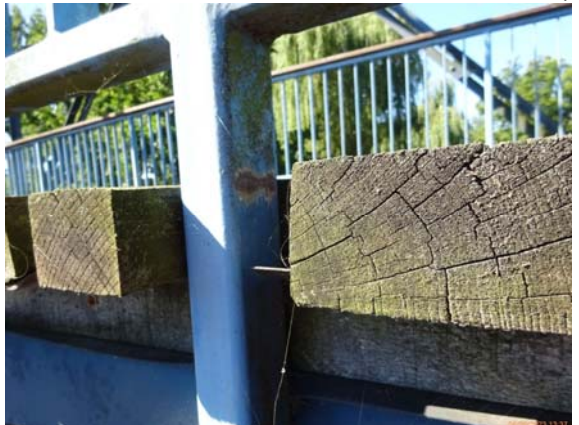
2023H-GEL - PFOSTEN ANGEROSTET
