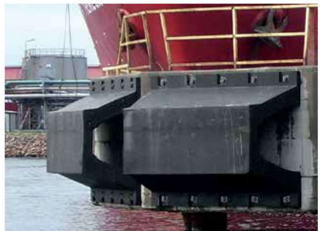
Turning Dolphin | Muuga | Estonia
